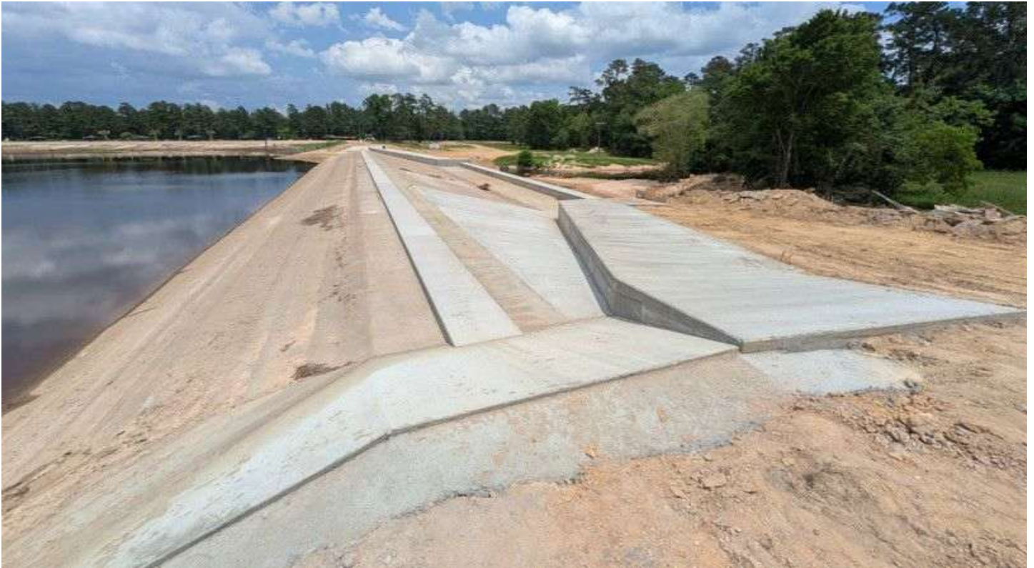
05/28/2025 - Repairs Complete & Cracks Sealed
