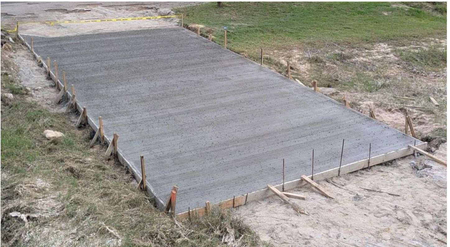
Boat Ramp Repair
